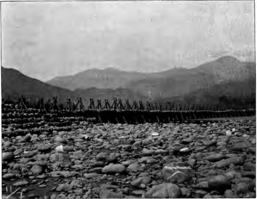
Near view of 'barrage' in position, shutting out the water from one of the two channels into which the river is here divided.
